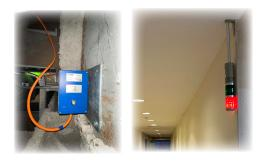
GeoSIG accelerometers (left) detect motion as part of the structural monitoring of the building. If the exceedance is deemed unsafe, red lights in the corridor (right) will alert people that evacuation is necessary.
